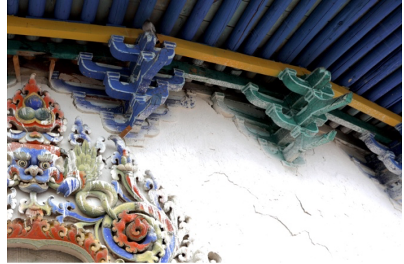
Fig. 4 Corbel Brackets under Roof of Bumpa, Gyantse Kumbum; Gyantse, Tsang region, central Tibet (present-day TAR, China); ca. 1427–1440; photograph by Shengnan Dong, 2021
